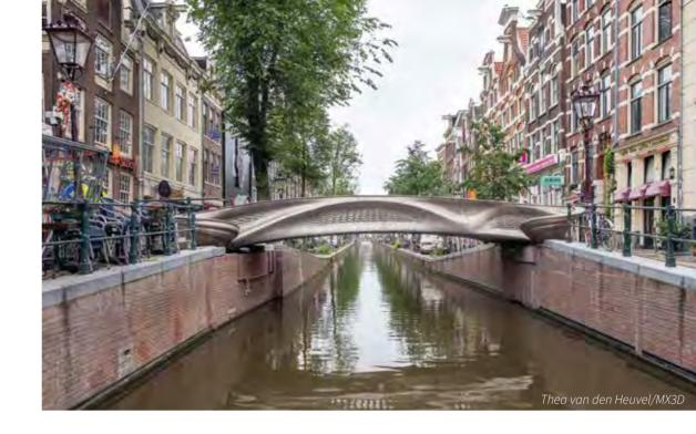
this pioneering structure. Support from Lloyd's Register Foundation allowed MX3D to tap into the Foundation's research network, bringing onboard partners such as ATI, The Welding Institute (TWI) and Imperial College, London. ATI carried out the data analysis to create the twin; Imperial undertook testing and helped design the network of sensors; and TWI was involved in devising guidelines for the production process. In addition, LR's quality assurance business assessed the system.
