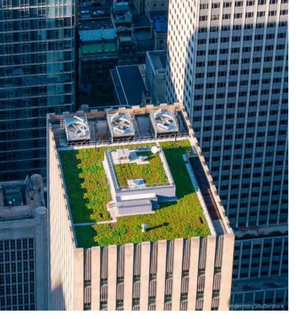
**ABOVE** The New York City government offers incentives to install green roofs that help absorb stormwater and prevent street-level flooding. Could infrastructure be designed from the outset to be more resilient in the face of disruption?
