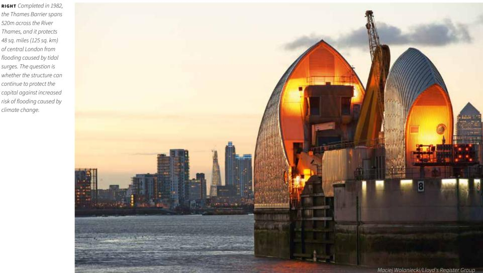
the Thames Barrier spans 520m across the River Thames, and it protects 48 sq. miles (125 sq. km) of central London from flooding caused by tidal surges. The question is whether the structure can continue to protect the capital against increased risk of flooding caused by climate change.
