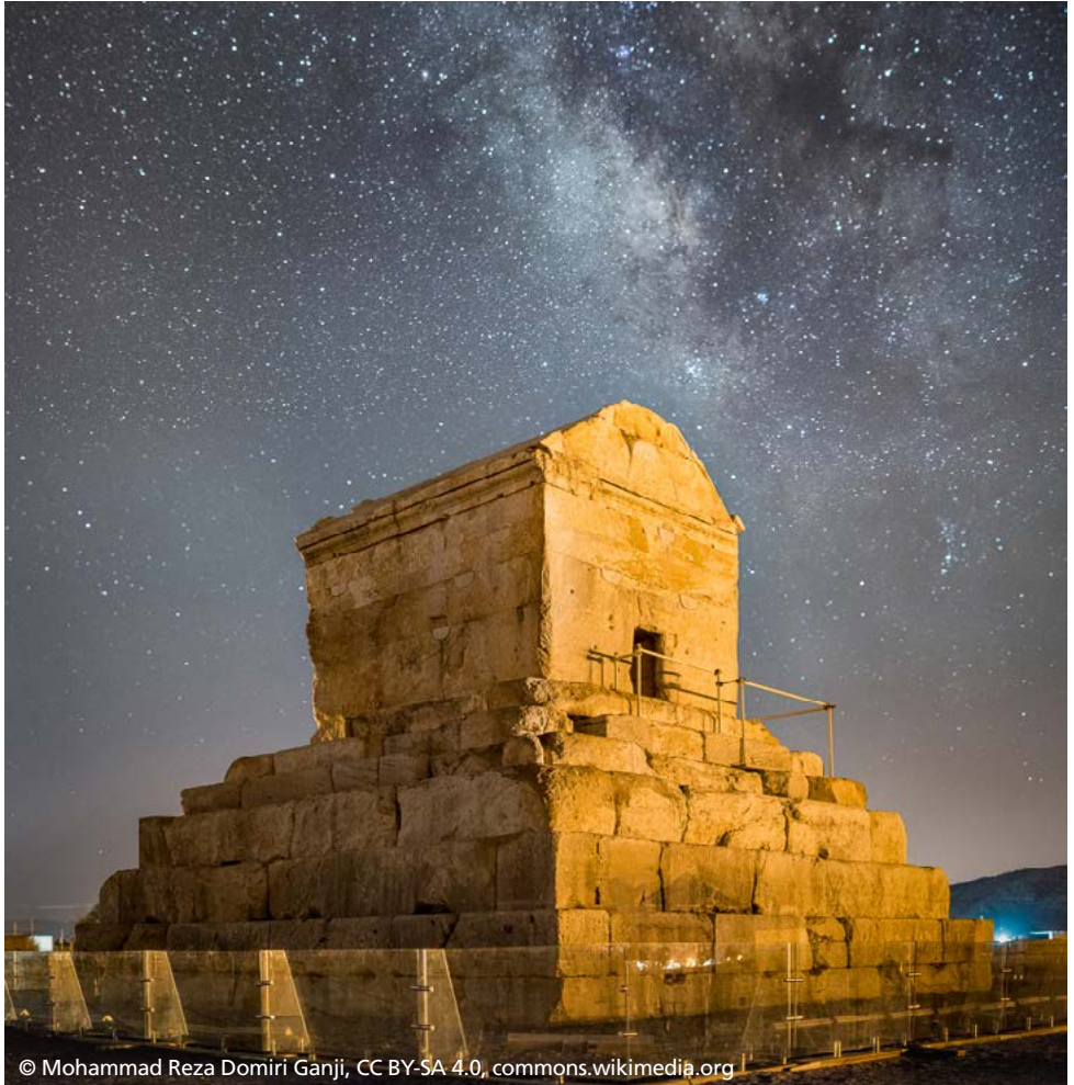
The Tomb of Cyrus, built in the 4th century BC, is said to be the oldest base-isolated structure in the world. Base isolation, also known as seismic base isolation, is one of the most popular means of protecting a structure against earthquake forces.
